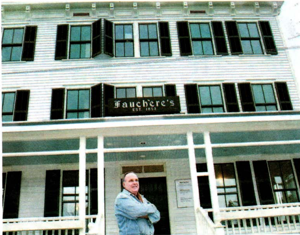
Mike Dilonardo, manager of the Hotel Fauchere in Milford, Pa., stands in front of the building last week. The hotel is going through a ground-up renovation aiming to draw high-end tourists to the area.
